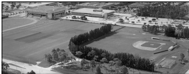
Kendall Campus Baseball Facility
